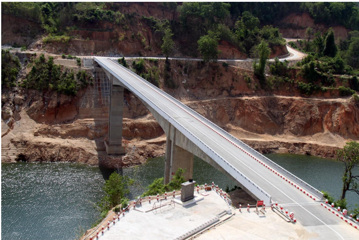
Photo : A newly upgraded Paletwa Bridge is underuse (1)
